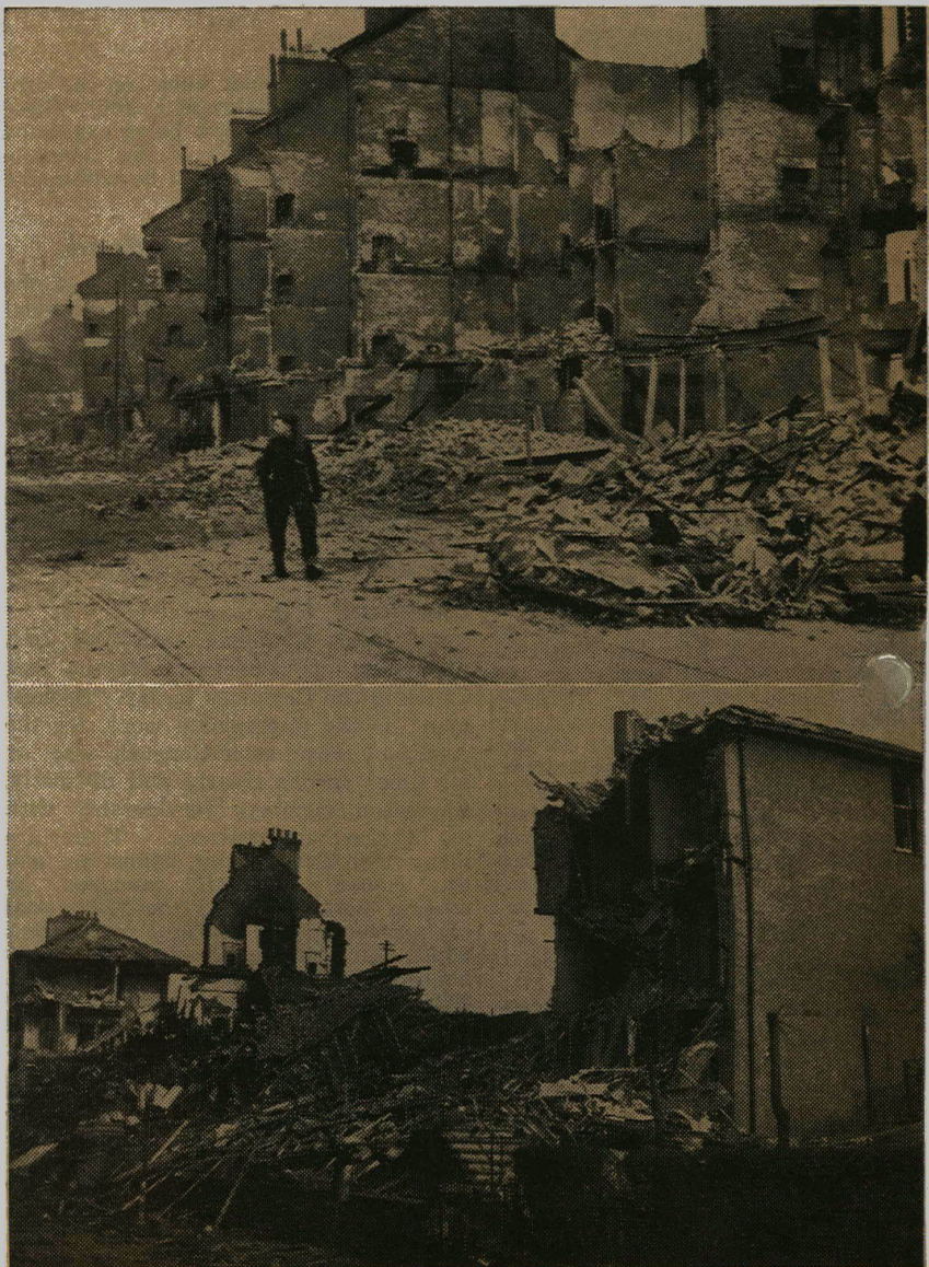
Tenement houses suffered most in last week's two-night bombing attack on Clydeside. The top picture shows a block of tenements, homes of working people, with the fronts completely blown out. In the lower picture the wrecked houses recall a scene in Ypres in the last war.
